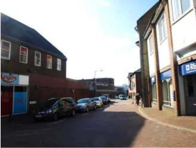
The wide splay of Drum Road leading south from New Rents reveals servicing areas with some blank facades and flat roofed buildings which have an adverse impact on the setting of the Conservation Area.
