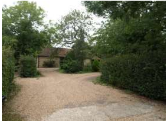
Mumford House (left) is set well back from the road and is well screened by hedge. The glimpsed two storey listed building comprises painted brick with a hipped tiled roof with chimneys.
